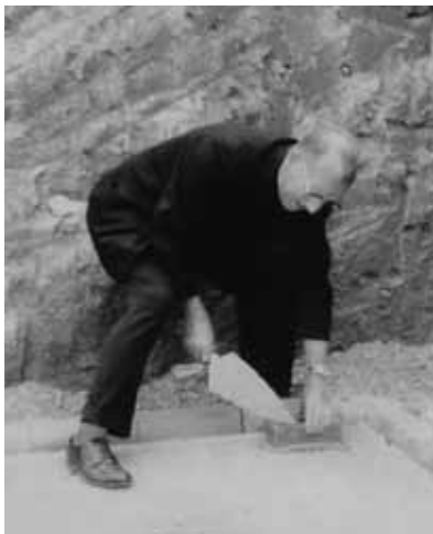
Father Murphy lays a brick in the corner of the new church.
