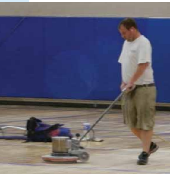
The gym floor was sanded, painted and sealed after last winter's flood.
